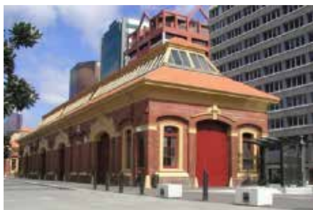
Shed 13, Queens Wharf
